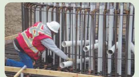
Assembling the rebar as part of the concrete foundation for a wind turbine. The foundation will eventually reside below the ground.
