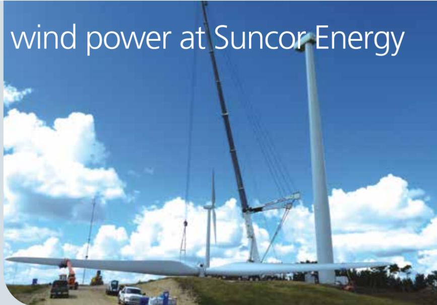
Lifting a 47.5-tonne rotor assembly into the air and onto the nacelle of a turbine.
